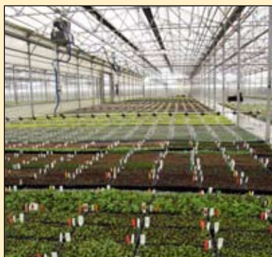
Automated watering system
