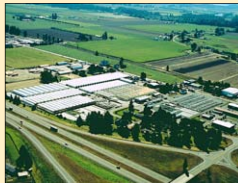
Skagit Gardens main location
